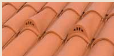
Hypothesis closure with traditional coppo-tile (instead cutting the DCS)
